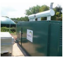
The new plant will provide 250kW of electricity, sufficient to power 450 homes, and 200kW of heat – so qualifying for payments from the government's Feed in Tariff and Renewable Heat Incentive programmes (14p per kW on electricity generated and 6.5p per kW for heat).
